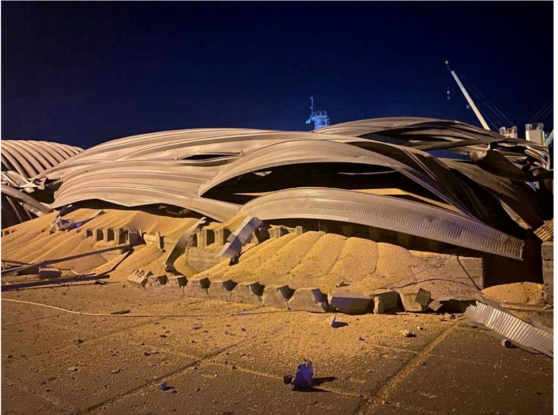
A grain depot at a river port on the Danube, Odesa Oblast, was destroyed on 16 August 2023.
